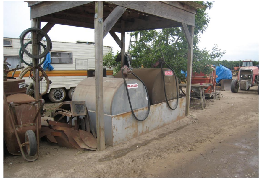
View of on-site ASTs labeled unleaded and dyed diesel fuel. Metal secondary containment is visible. Liquid is noted within secondary containment.
