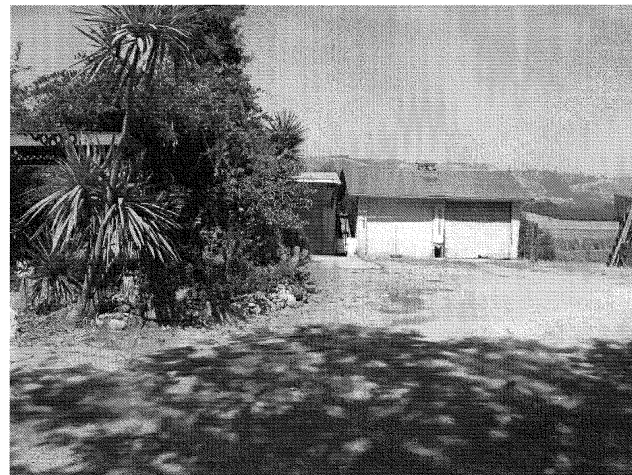
3. View of the garage attached to the southeast side of the residence.
