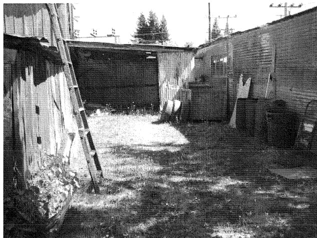
6. View of sheds, tires, and empty plastic drums in the southwest corner of subject property, with PG&E substation in background.
