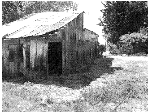
7. View of sheds southwest of the residence.
